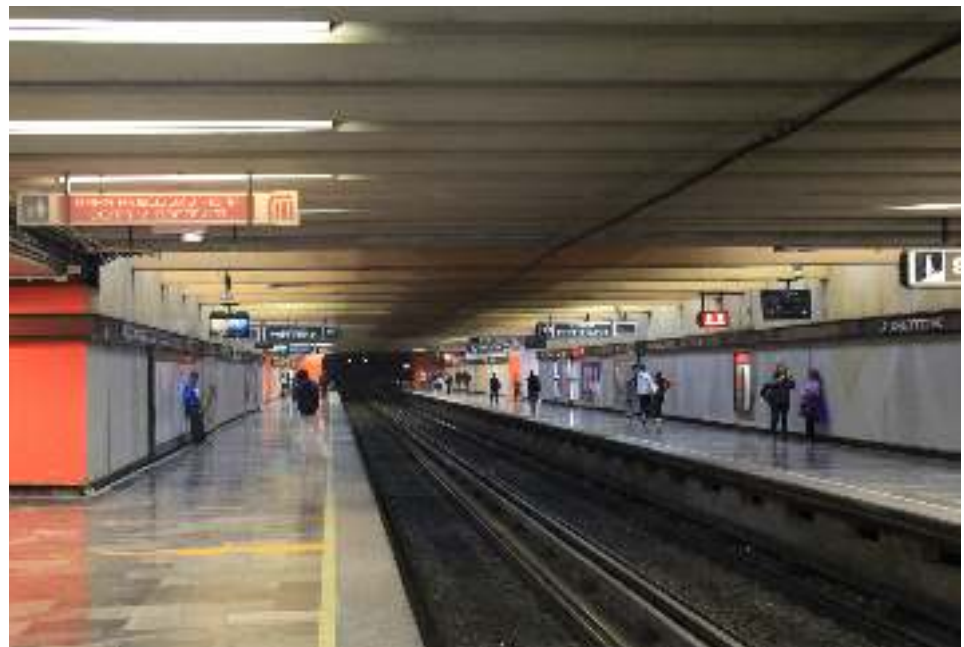
Chilpancingo metro station. Credits: Franck Giraud.
