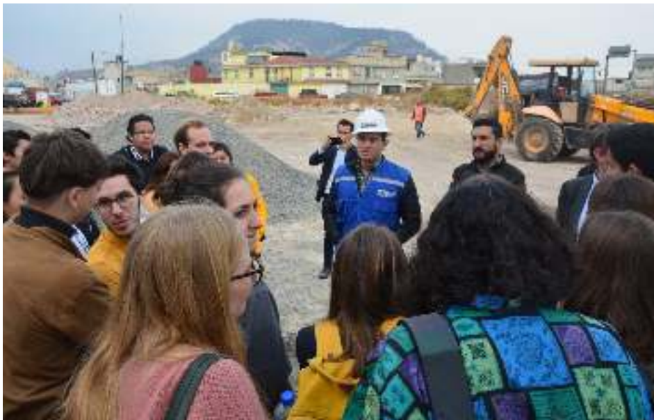
Field visit of the Mexico-Toluca City Train construction site. Credits: Anouk Jeanneau
