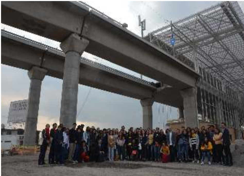
Field visit of the Mexico-Toluca City Train construction site. Credits:Anouk Jeanneau
