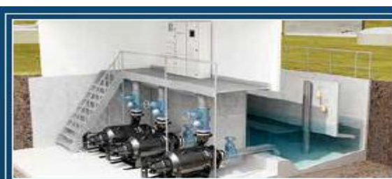
5 pumps can be used for dry installation when fitted with cooling jackets.
