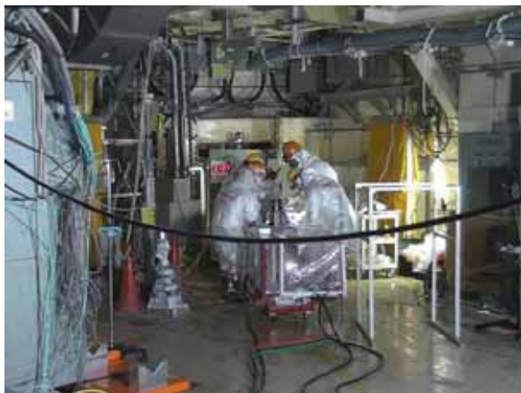
Work outside the PCV (In front of X-6 penetration)
