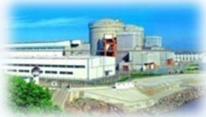
Construction of 650 MWe NPP CNP600
