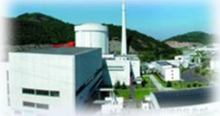
Construction of the 1st NPP (300MW PWR)
