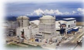
Construction of CNP1000
