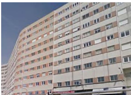
Painted concrete façade
